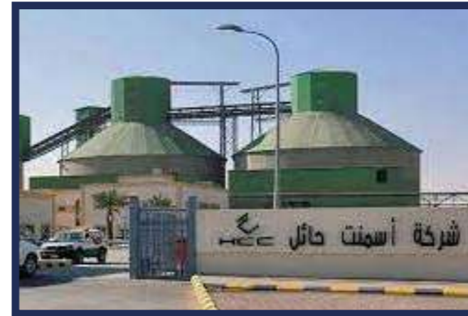
Hail Cement Factory
